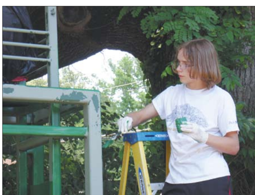
Nicholas West worked on earning his Eagle Rank with Boy Scout Troop 506 in Halls - Knoxville by refurbishing the main gate at Fountain City Park as well as sanding and painting two bridges that enter the park from the Broadway.
