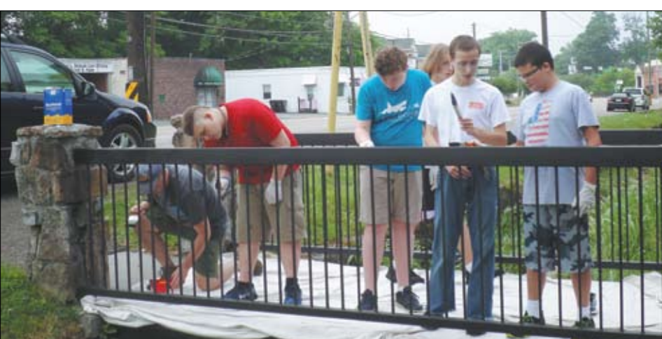
Eagle Scouts David Denton, Braden Mast, Ryan Howard, Jonathan West, Nicholas West and Zarian Stephens paint one of the two bridges leading into Fountain City Park.
