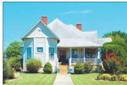
2849 RENNOC ROAD Knoxville, TN 37918
