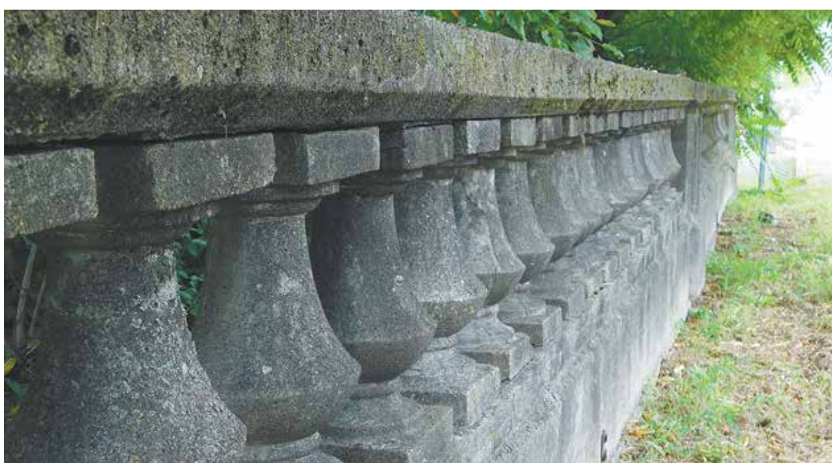
The odd pillars of the walls above the Mineral Springs Bridge and the two arches below make the old span beautiful and historic. Built in 1910 as the area was developing as an entrance to the historic Whittle Springs resort area, the new bridge is longer but may resemble the current one a bit.
